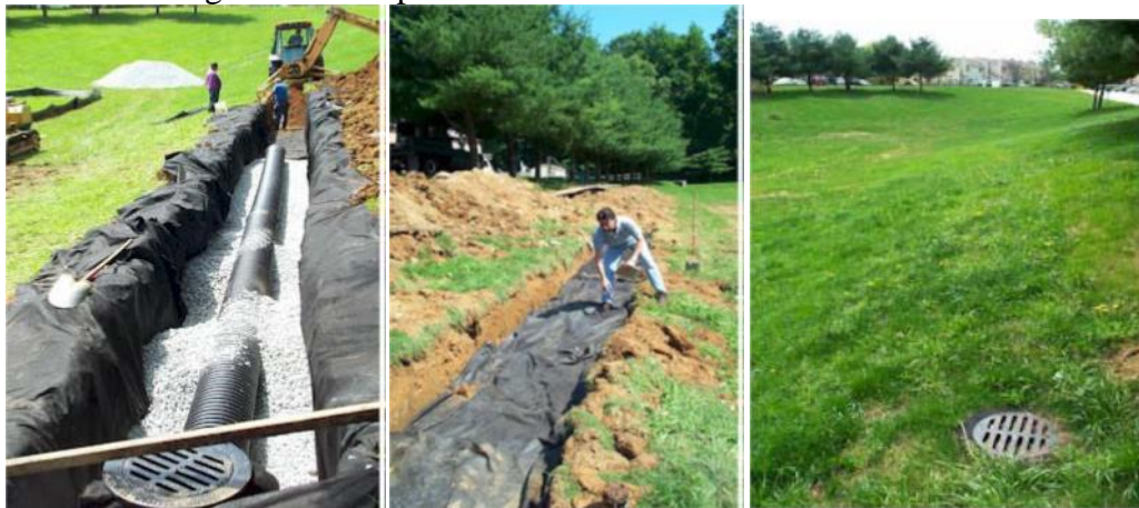
Figure 4: Example of Infiltration Trench Installation
